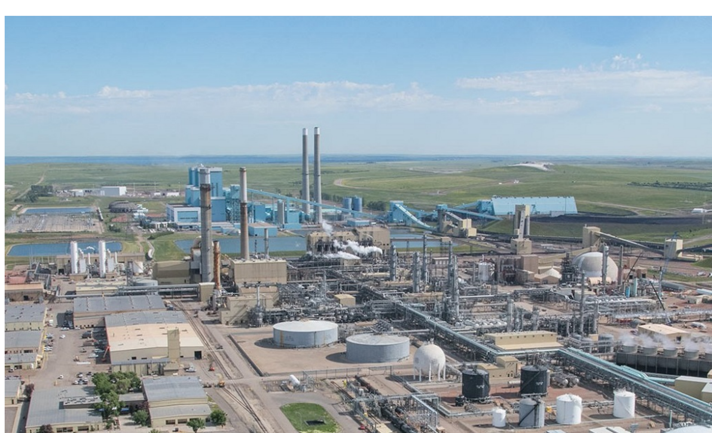
The Great Plains Synfuels Plant near Beulah, N.D., is the only commercial-scale coal gasification facility in the United States that manufactures natural gas. Dakota Gasification Co. photo.
