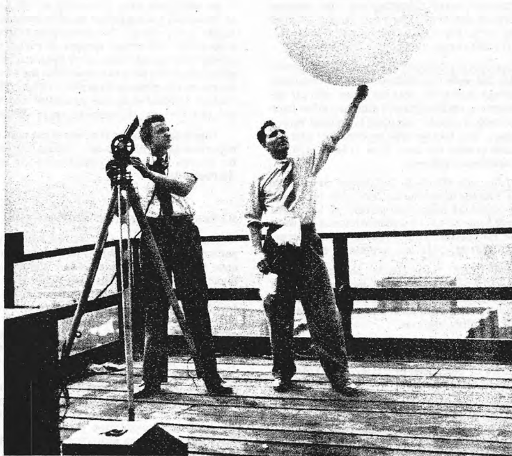
Fig. 7 Radiosonde balloons carrying baskets of solid carbon dioxide into the upper atmosphere
